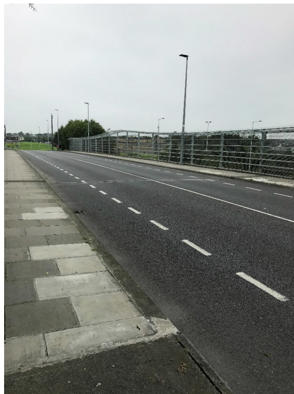
Photo 2 – Existing Greenhills Road Bridge looking west
