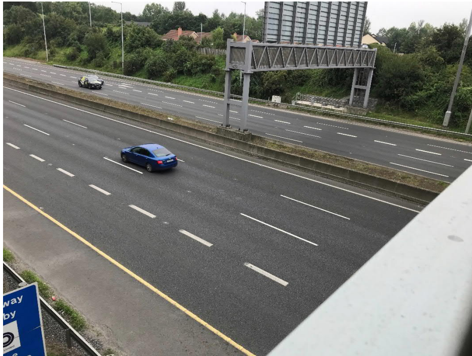
Photo 1 – Proposed bridge location spanning the M50
