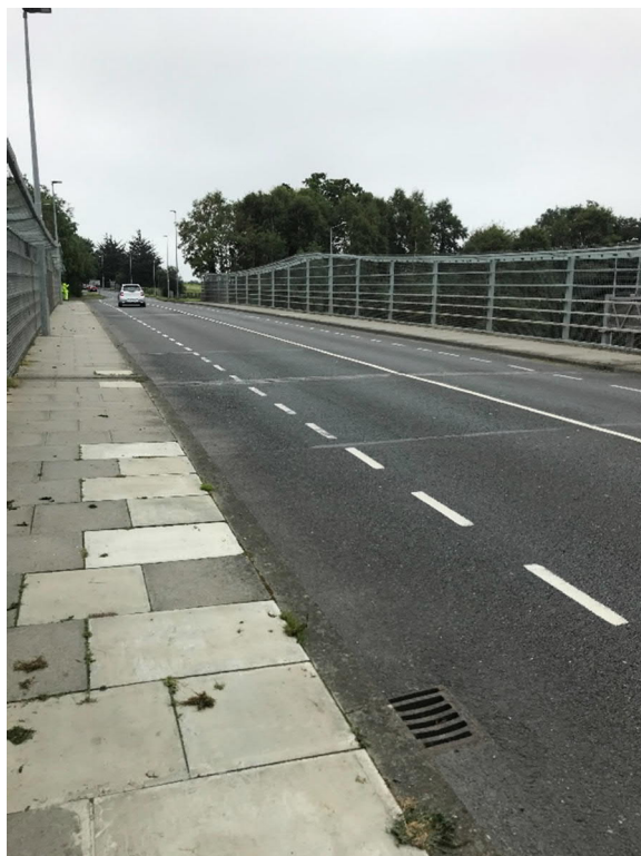
Photo 3 – Existing Greenhills Road Bridge looking east
